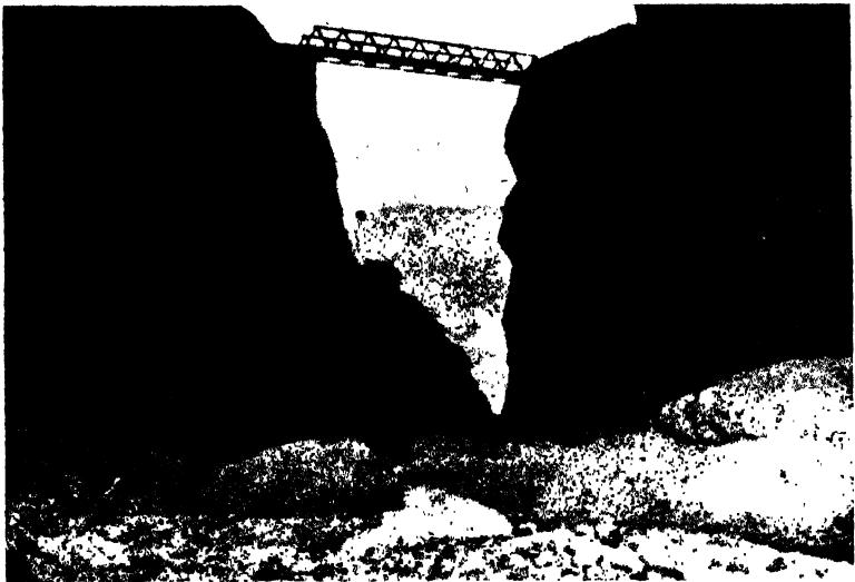
CHAPPAR BRIDGE. View from the other side.
