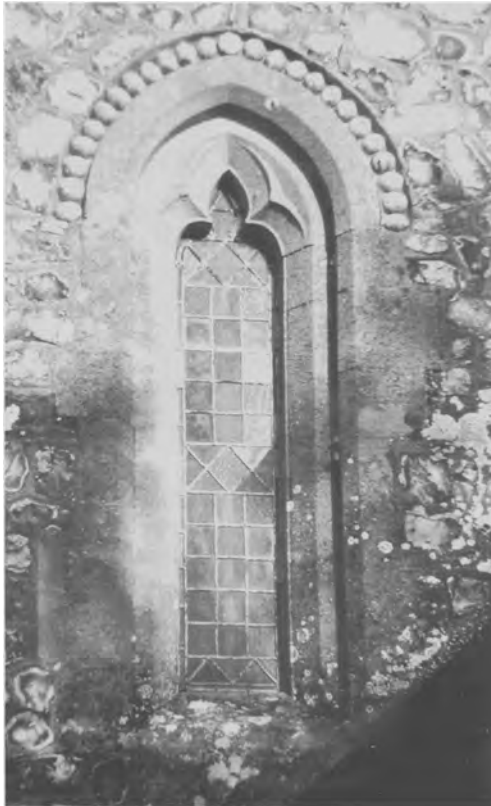
Fig. 8. Nineteenth century window on south side of St Peter's church, Linkenholt, framed by fossil echinoids.
